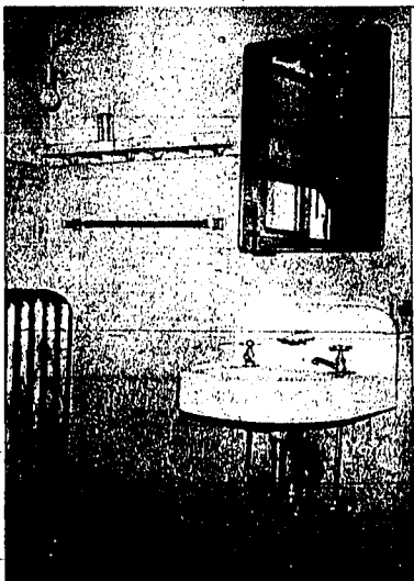
PLUMBING AND HEATING present problems in the new Harbor House in Twin Falls. Much of the wiring must be re-installed and Civitan Club members have offered to assist with this and other projects. This utility-bath room on the first floor is in for some changes.
