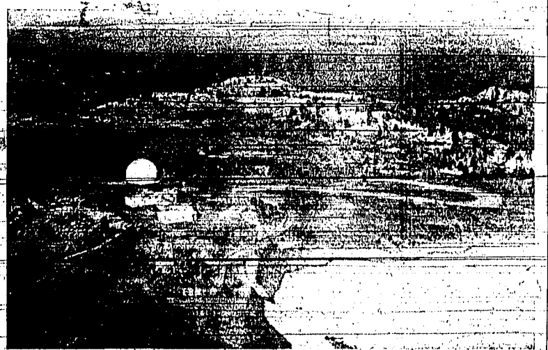
RADAR BUBBLE IN the McCall area lets human scanners in Salt Lake City know exactly where various airplanes are operating... Stations throughout the United States, blanketing the United States. In the west, although pilots feel they are flying over miles of nothing, they are seldom out of sight of radar.
