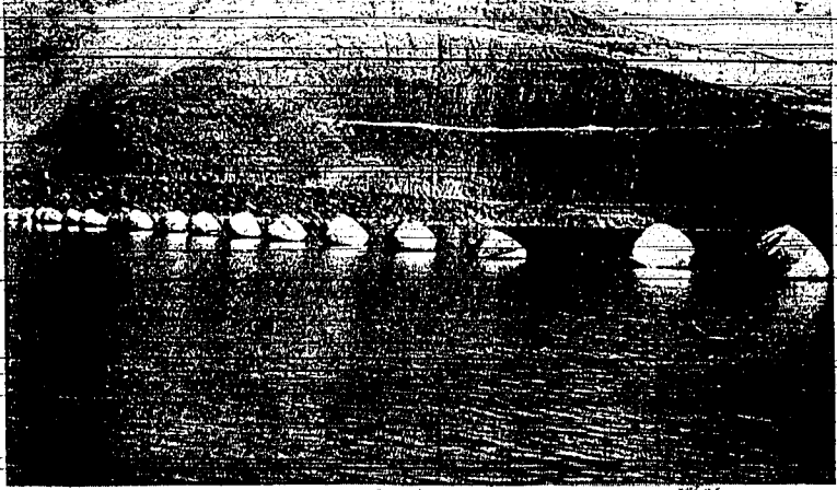
FLOATING METAL BARRELS, anchored together, are a warning to boaters to stay out of the area between the obstructions and the dam. The Hells Canyon area, at all three
