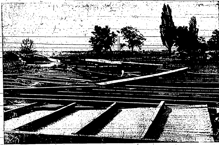
ONLY FLATTENED BOARDS remain of what was an aluminum storage shed at the Jerome Country Club until it was demolished by a freak windstorm Saturday night. The building was lifted from its foundation and carried several hundred feet. Dick Lowe, manager of the club, said the wind
