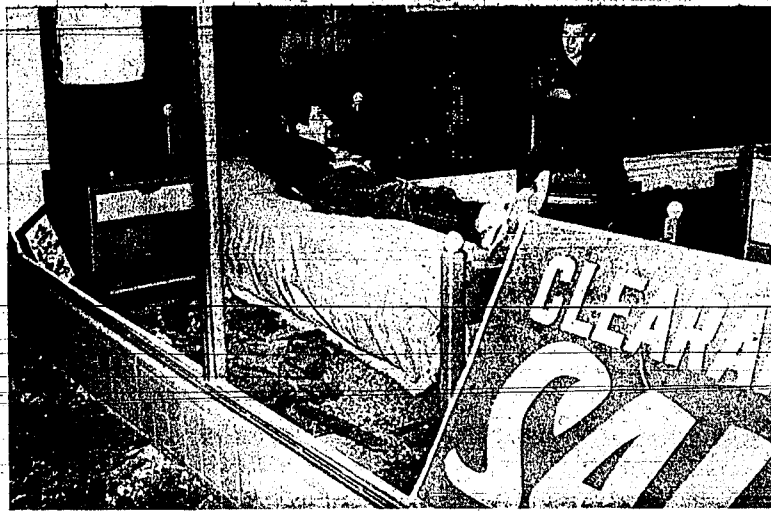
AFTER A SERIES of sharp earthquakes late Wednesday demolished most of the plate glass of the Santa Rosa Furniture Co., these two young men kept an all-night vigil to prevent looting. Van Nielsen, the owner's son, right, chats with
