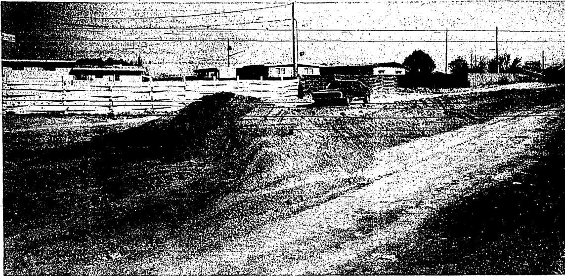
CONSTRUCTION WORK IS continuing on the portion of Falls Avenue from Harrison Street to Blue Lakes Boulevard North. The city is now widening the street, but motorists are still traveling on the far sides of the street. Jean Miller, acting city manager, said the biggest part of the work will be completed this fall. A temporary surface will be laid this fall and the permanent surface will be put on when warm weather permits next spring. The Falls Avenue work will continue as long as the weather allows.
