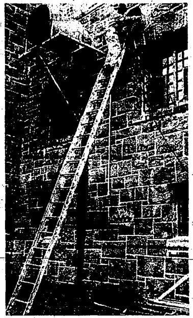
A WORKMAN WELDS steel bars into the opening of a 2 1/2-foot ventilation duct at Rocky Butte Prison near Portland after five prisoners crawled through and dropped feet to the ground to make their escape on Monday. Tracks indicated the men made their way across the prison compound, climbed a fence and fled. (UPI telephoto)
