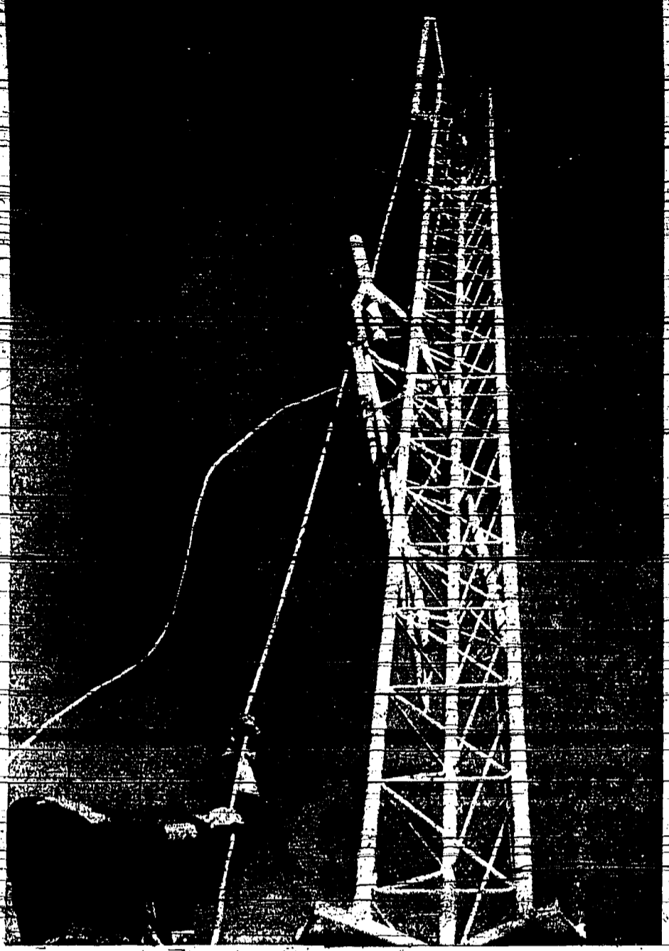
THE FIRST STEP IN A modern radio emergency communications system at Magic Valley Memorial Hospital was finished when this 56 foot antenna was put into place on top of the hospital. At the top is Bob Bailey and at the bottom of the picture is Terry Williams, both technicians for Technical Electronics Corp. of Twin Falls. The antenna will be hooked to a power base station in the hospital and eventually physicians in the area will be able to be paged in their cars or at home by use of this modern radio system. The system costs about $5,000 and was donated to the hospital by members of the Magic Valley Memorial Hospital Medical Staff. The system consists, at the present time, of the antenna and base station.
