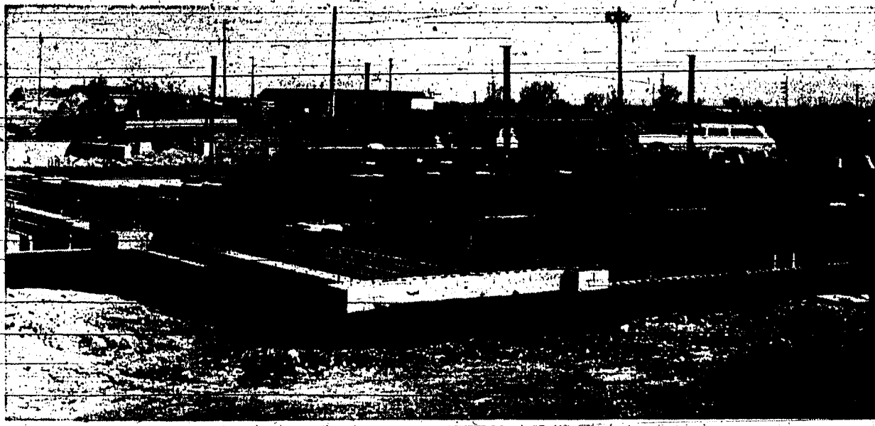
OTIS HALL CONSTRUCTION Co. is on schedule with its work on the new Child Development Center. The building is being constructed on Harrison Street, just south of the
