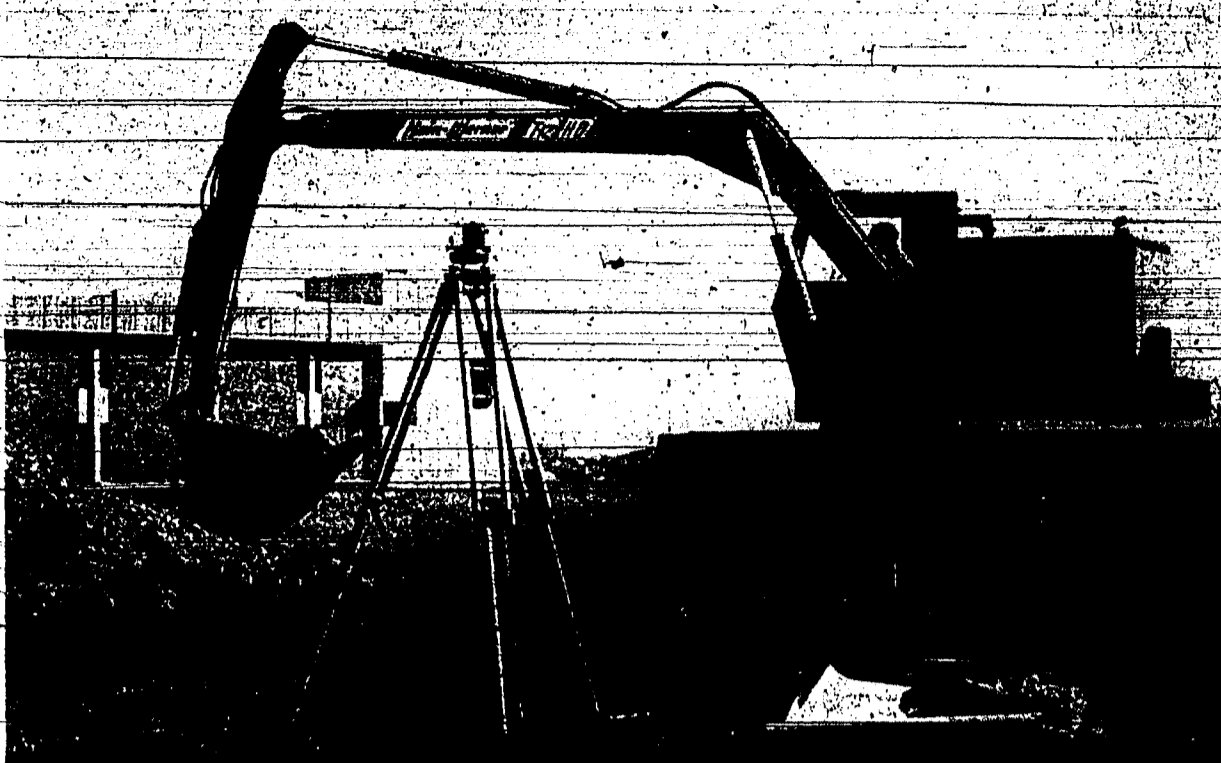
GROUND WAS BROKEN last week at the site of the College of Southern Idaho "commons" by Nelsen and Miller Construction Co., Twin Falls. This far this back hoe is the only large piece of equipment on the site, just east of the Fine Arts Center. In the foreground is a transit which project engineers are using on the site, and at the right of the photograph are the project plans. Nelsen and Miller, which
