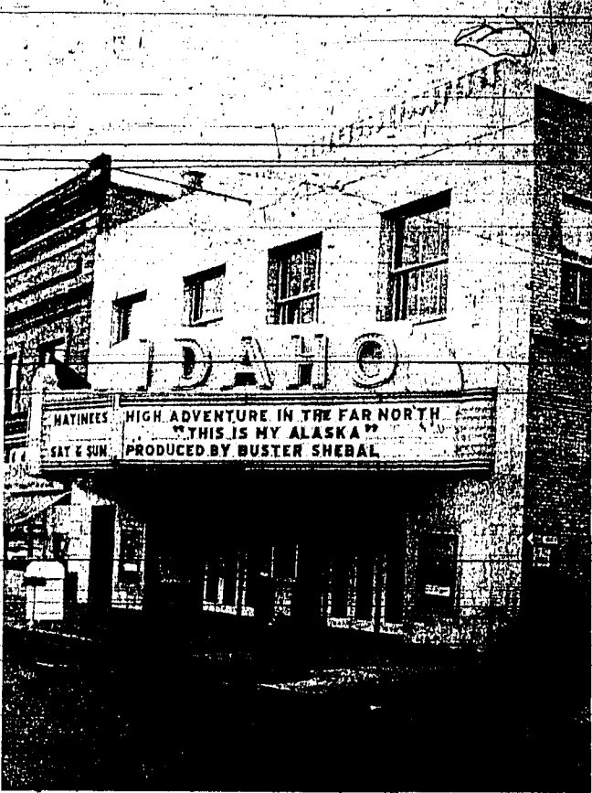
THE IDAHO THEATRE building will be demolished sometime in February as part of the Twin Falls downtown improvement project. The structure, built in 1915, was purchased recently by the Twin Falls Urban Renewal Agency. The property will be offered for sale at a public auction. James Kelsch, executive director of the agency, said it is hoped another building will be erected on the location.
