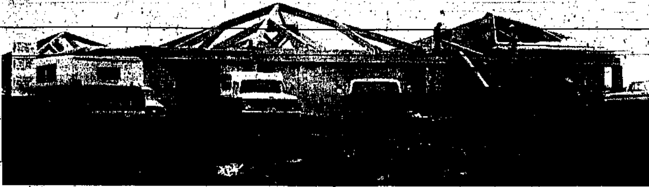
CONSTRUCTION OF THE Child Development Center on Harrison Street is progressing on schedule, according to director Paul Burnett. The building, under contract to Otis Hall Construction Co., will be completed in May or June. The center office is now located in the old gynecologist's office at Magic Valley Memorial Hospital. In the meantime, activities of the center are continuing, with students of varying ages enrolled in a number of self-help programs designed to increase coordination, develop maturity and inspire self-confidence.
