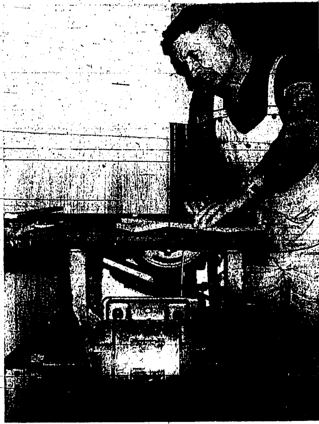
ONE-OF-THE-CARPENTERS working on the remodeling of state offices at the Maladok LDS Tabernacle in Rupert, is Ed Anderson, Burley, who here is busy at the table saw where wall paneling is being trimmed to fit the hallways.
