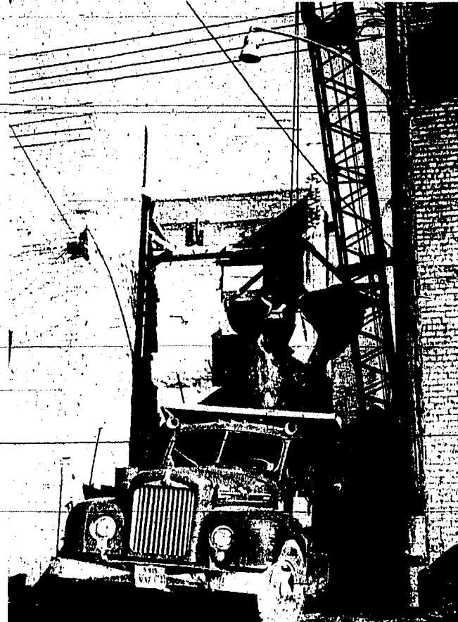
WALLS OF IDAHO THEATER building are coming down in the current Urban Renewal project to remove sub-standard buildings. Under contract with the Northwest Rigging and Crane Co., the work has been under way the past two weeks. All that remains of the old theater and office building are the exterior walls and overhead beams. Trucks are hauling away the brick from the rear wall and expect to be working on side walls this week.
