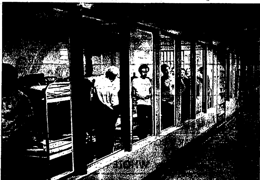
BARNS HAVE BEEN replaced with plate glass windows in the reception wing of San Diego County Jail, Calif. Less fire-bidding than bars, they nevertheless provide equal security.
