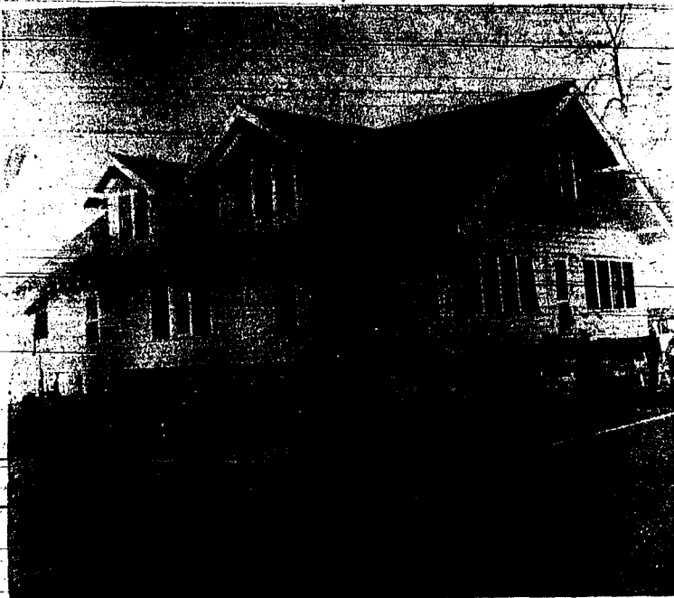
MOVING A TWO-STORY HOUSE FROM a residential location near downtown Twin Falls to a semi-rural location on the Northwest edge of the city is no easy task. The size of the house here indicates just what kind of job it will be. The house, at 120 Sixth Ave. N., will be moved next week and in 60 days will become the home of Walt Blaylock. He purchased the home
