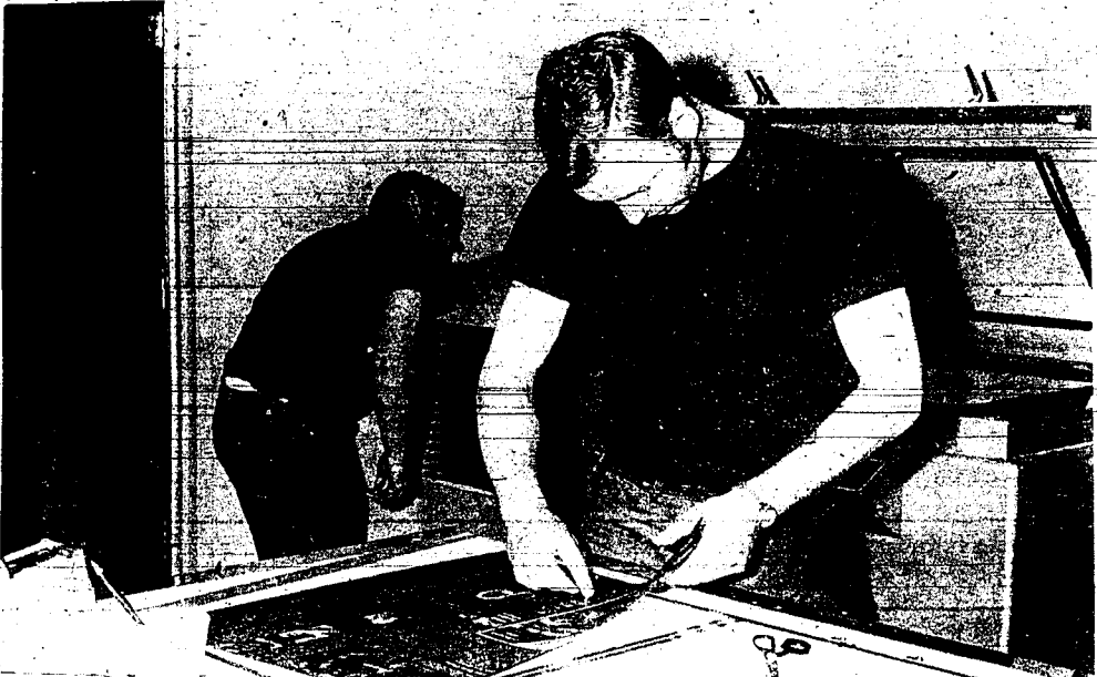
EXAMINING a page negative, a negative which will be used to make a photograph on a metal plate and later placement on the press—News. Behind him is Al Mingo— is Jack Tucker, a pressman for the Times—
