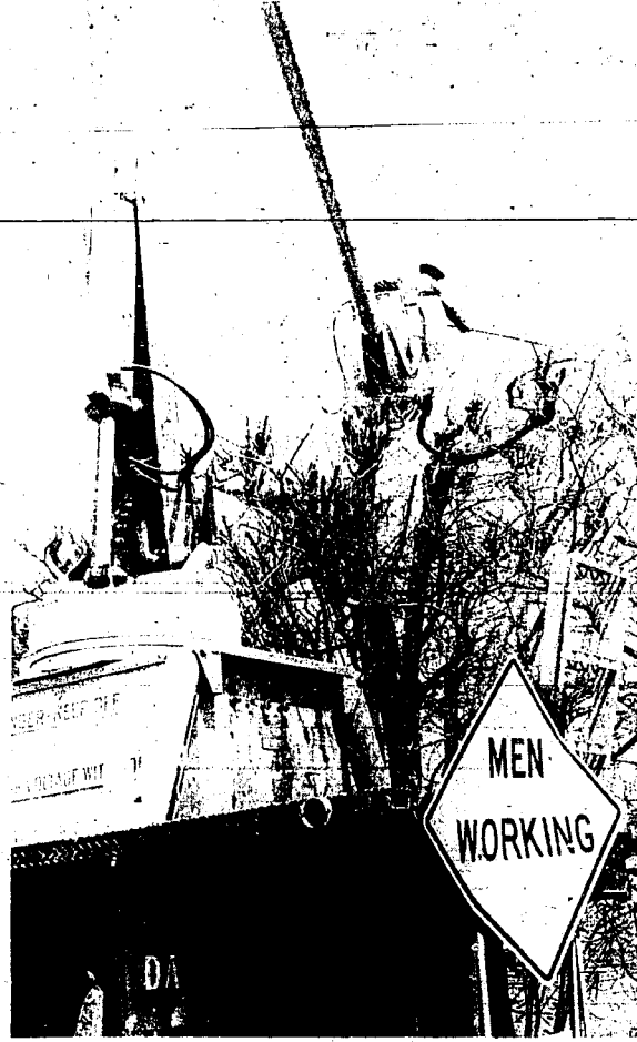
RIDING HIGH ON a boom mounted on one of the company trucks is a workman for Davey Tree Service. The firm is contracted by Idaho Power to keep power lines clear of branches. This week the men and equipment were working in the area northwest of Twin Falls.
