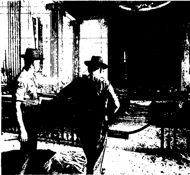
STATE POLICE LOOK over the damage from a bomb to the Louisiana State Capitol Monday. A bomb exploded in the Senate Chamber of the skyscraper State
