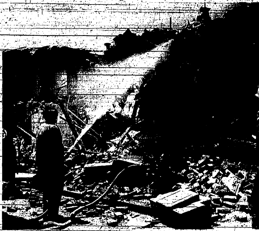
A FIRE HOSE MAY seem like a strange accompaniment for a demolition job, but it helps to keep the dust down. A crew tearing into the building housing the former Salvation Army Thrift Store at Third Street and Main Avenue East Thursday used a fire hose hooked up to a fire hydrant to wet down the debris, while a crane-mounted grabber bit huge chunks out of the wood-and-brick structure. The demolition is part of the continuing first phase of urban renewal. A parking lot will replace the building until the downtown mall gets under way.
