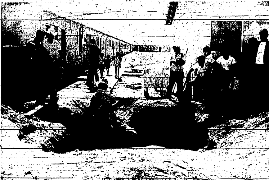
MIGRANT WORKERS at the new labor camp east of Hammett, in Elmore county, help build a sprinkling system to water lawns which will be planted at the camp. The four buildings, each containing 12 or 13 units, are located in a square, and the open space in the middle is being made into a recreation area with playground equipment planned. One of the amenities of the camp is the coin operated washing machine, in addition to electric stoves, below. Each living unit has refrigerator and hot water.
