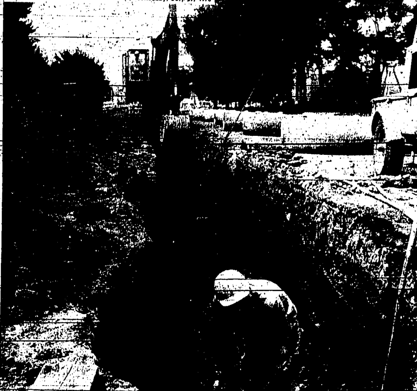
TRENCHES ALONG SHOSHONE Street in Twin Falls are being dug for installation of a storm drain line to carry rain and melting snow water from the downtown area. City officials said work will progress one block at a time, with the block involved in the work being closed to traffic. Here, Neilson and Miller con-
