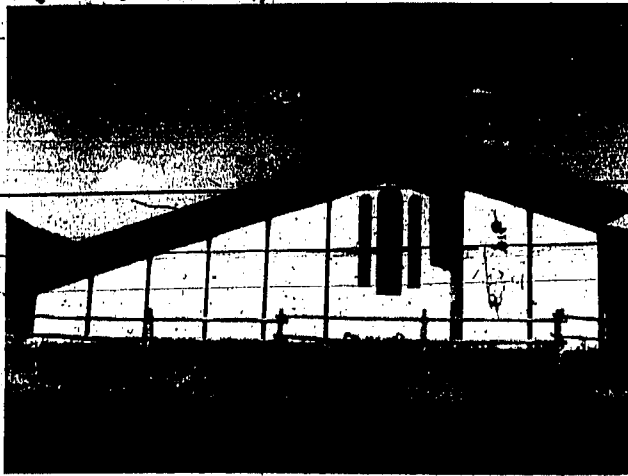
KETCHUM AND SUN VALLEY'S newest church, Our Lady of the Snows, will be dedicated Sunday with Bishop Sylvester W. Treinen of the Catholic Diocese of Boise, officiating. The newly-constructed church features several interesting items, including a 12-foot Italian carved wood statue of the Madonna, as noted in this photo.
