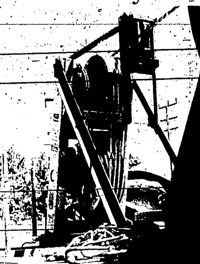
AT THE OTHER end of the mile-long project, wire from the 4,900-foot supply reel is fed through a "tensiometer" device to produce a constant tension over the entire length of wire. Each reel of wire weighs nearly a ton, and linemen are kept busy jockeying the reels as the wire is fed through the pulleys and onto the poles.
