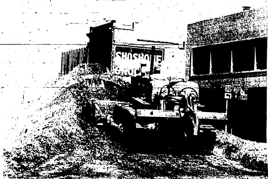
AS SURGEONS must cut to repair the human body, so these "civic surgeons" must make a mess out of the Twin Falls downtown street, as a part of the development program. This pile of dirt on Main Avenue is part of the mall project which is moving rapidly toward conclusion — chairreuse sidewalks and all. In the first blocks to be torn up, the rebuilding is taking firm shape. (Times-News photos by Dan Johnson)
