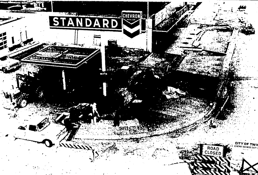
AN AERIAL VIEW of the downtown redevelopment project shows the beginnings of some form as sidewalks and curbs are poured. The project is moving along rapidly under favorable weather conditions.
