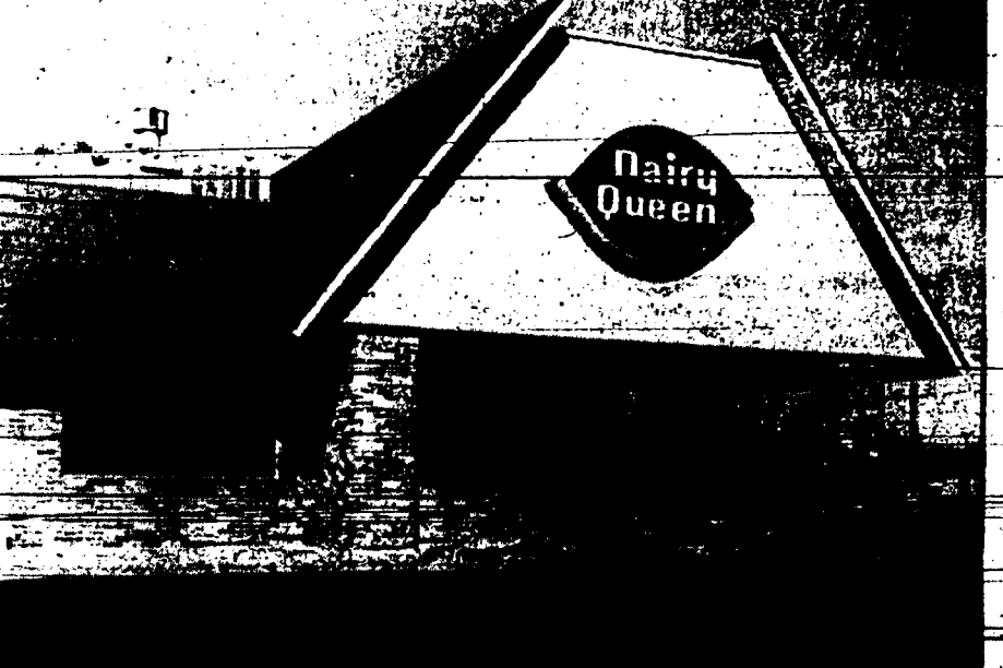
NEW BRICK STRUCTURE at 2200 Overland Avenue, Burley, houses the Dairy Queen which is now open for business. Mrs. Alice Haycock, manager, said a grand opening is planned for
