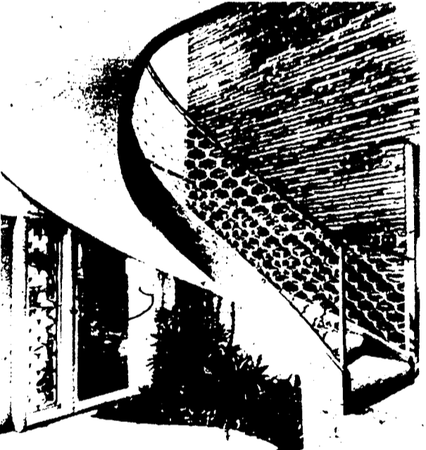
MODERN ALL THE WAY. The handrailing of this contemporary stairway, with its gracefully sweeping curve, is accented with a decorative, yet simple, pattern of stock ornamental castings.
