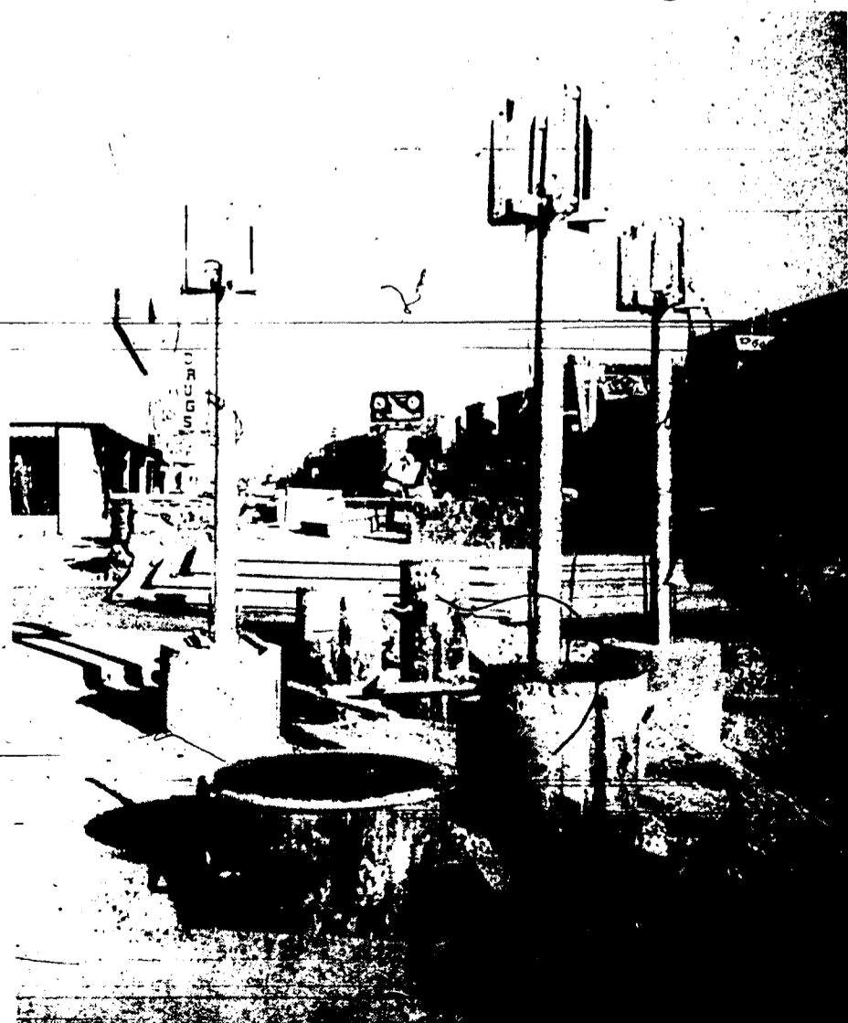
EARLY "PLANTINGS" in new downtown Twin Falls scene include these electrical fixtures which will become part of the mail block. Work is nearing final stages in initial two blocks and shoppers and business owners are beginning to get an idea of what it is all about. Rock retaining walls and elevated area will provide rest area and traffic protection for pedestrians.
