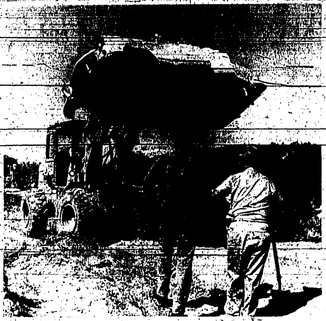
OLD CAR BODY; soon to be crushed and shipped out as scrap metal, is used here to add weight to equipment packing down new dirt over the culvert installed in Rock Creek Canyon just west of the hospital. The crossing was completed Wednesday and will allow crusher equipment to move into the canyon and begin clearing away junk cars now littering the Rock Creek site. Fred Radcliffe, left, directs the operation.
