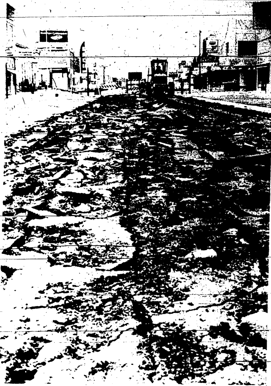
Freshly laid asphalt in the first block on Main Avenue West didn't meet specifications. It was promptly ripped up and replaced.
