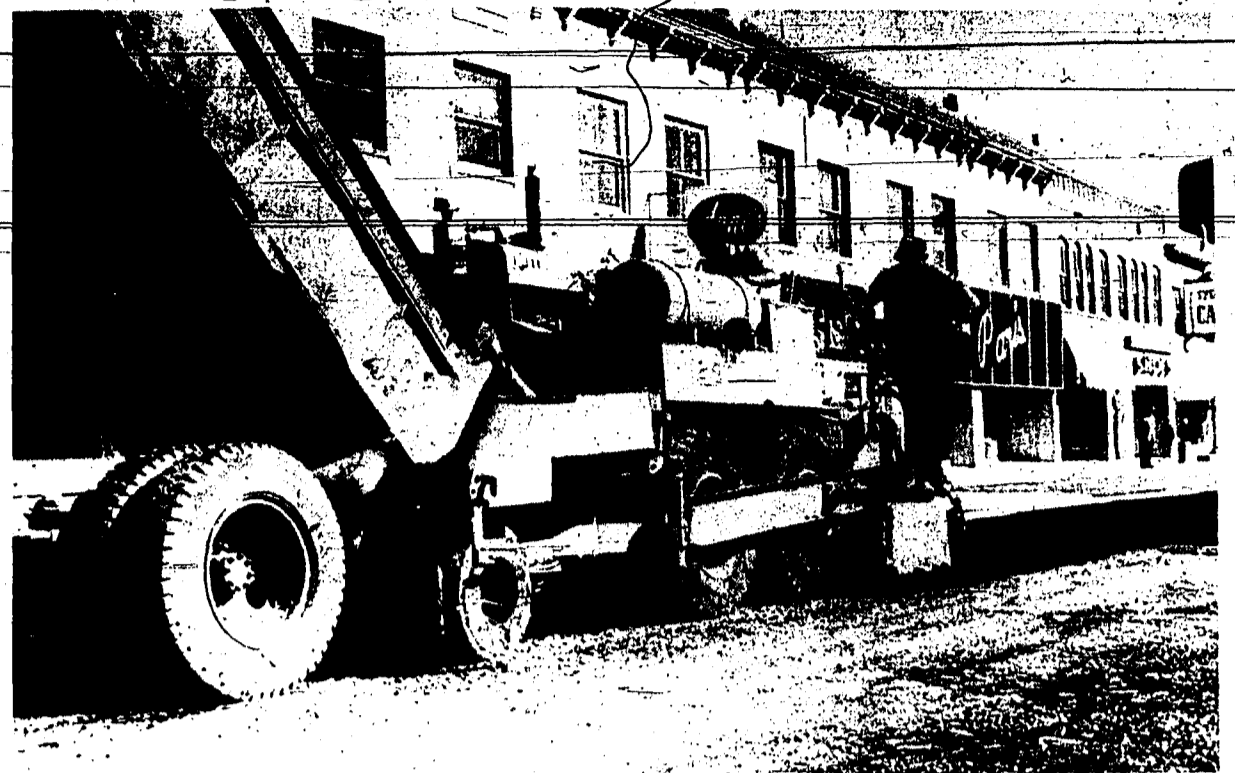
Assorted heavy equipment was used in mall construction work, including graders, left, and paving units, below.
