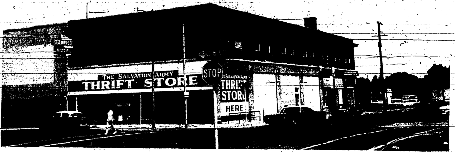
With the snows of yesteryear is this brick structure, which one stood at Main and Third Street East.
