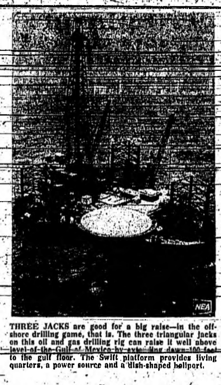
THREE JACKS are good for a big raise—in the offshore drilling game, that is. The three triangular jacks on this oil and gas drilling rig can raise it well above level of the Gulf of Mexico by as much as 100 feet to the gulf floor. The Swift platform provides living quarters, a power source and a dish-shaped heliport.
