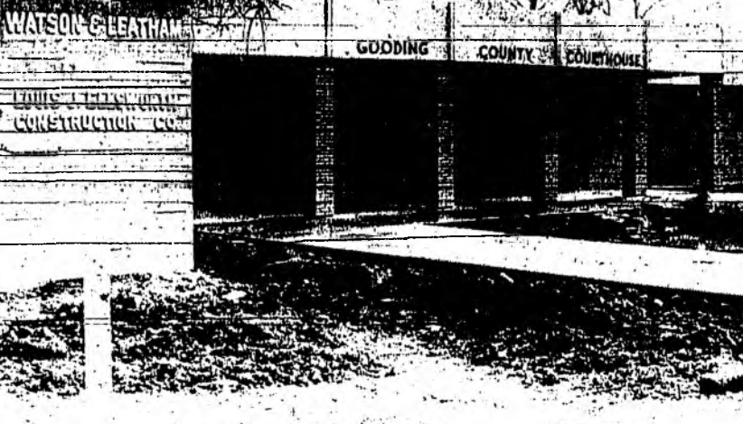
Courthouse . . . COMPLETION OF THE new Gooding county courthouse is scheduled for January. The structure, being built by Louis J. Ellsworth Construction Co., Blackfoot, is located on Main Street. The contract is for $318,000. Subcontractors were First Street Plumbing and Heating, Idaho Falls, and Cook Electric, Twin Falls.
