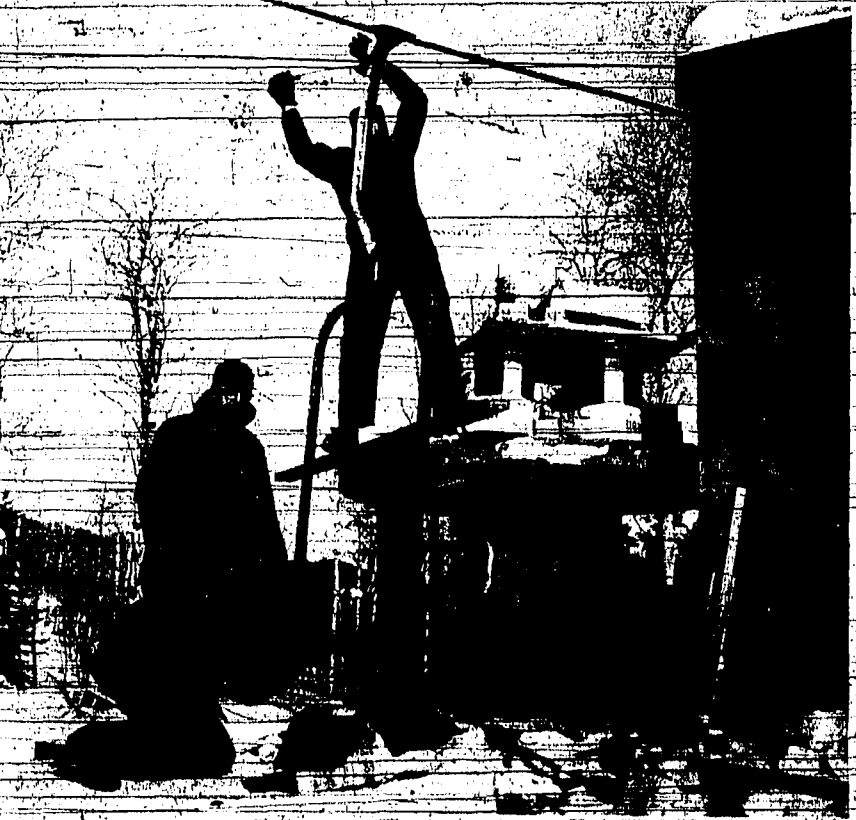
Chair lifts . . . ONE OF FINAL STAGES on construction on a new double chair lift at Magic Mountain was completed this past weekend as construction workers attached chairs to the cable. Ed Berg, top, fastens the ball structure of the chair to the cable, while co-workers attach the seat framework. The new lift is expected to be in operation within the next two weeks.
