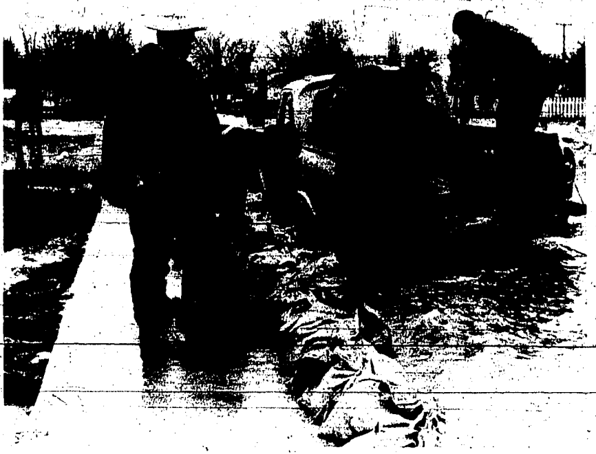
SANDBAGGING in Jerome continues today. Here city crews are busy sandbagging Sixth Street East to prevent water from running over the sidewalk onto private property. Homes along Sixth Street West and North Date Street were flooded today from an overflowing coulee. (Photo by Charlotte Bell)
