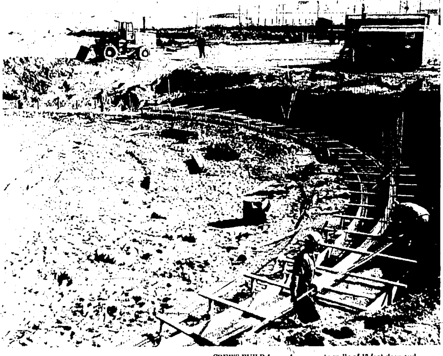
CREWS BUILD forms for concrete walls of 13-foot deep and 115-foot diameter clarifier at the Ore-Ida Foods' secondary waste plant being constructed at the Burley plant. Nelsen-Miller Construction Co., Twin Falls, is contractor for the project.
