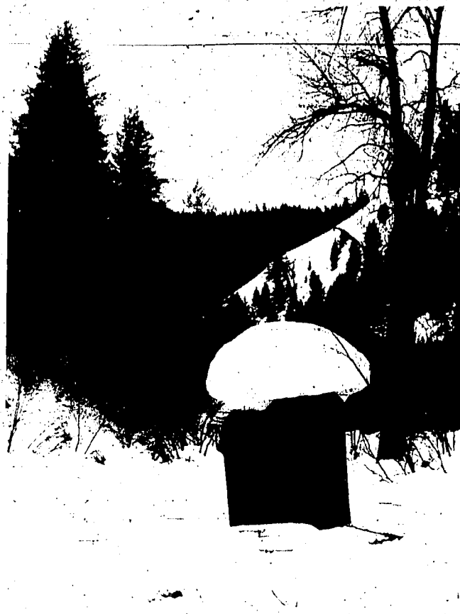
SNOW TUFT SPORTED by this rustic facility tells the story of weather conditions in the Warm Springs area above Ketchum. While most structures have been cleared to prevent roof damage, someone apparently forgot about this important building. (Photo by Larry Hovey)
