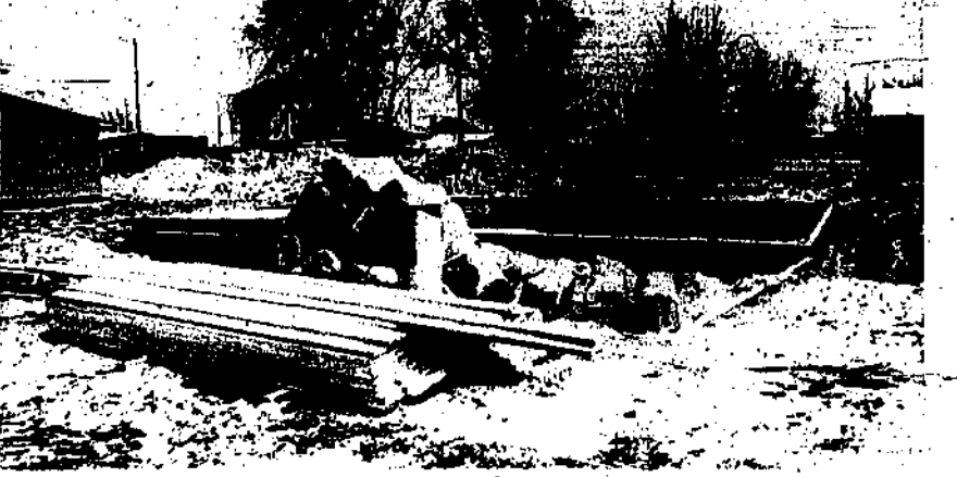
SNOW COVERS building material! on site of one of 12 houses at Paul being built by Dale Milton ContrucUon Co. Seven homes are complete and other* are expected to be uUha M days.
