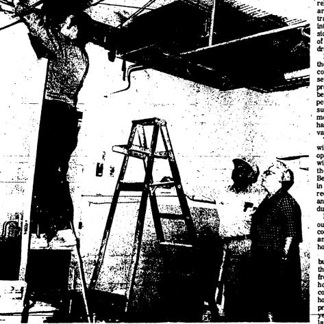
Duct work - FOUR-BED WARD on the fifth floor of Magic Valley Memorial Hospital is temporarily out of service while air conditioning equipment is being installed. Here Hospital Administrator Irene Oliver and work foreman Dorsey Miller watch workman installing cold air duct.
