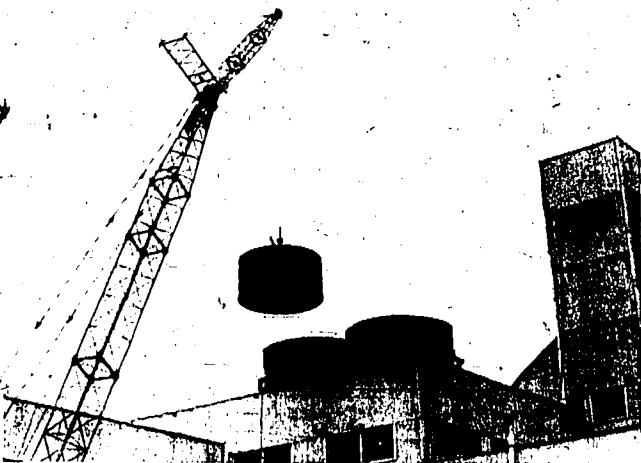
First step in installation is hoisting units into place
