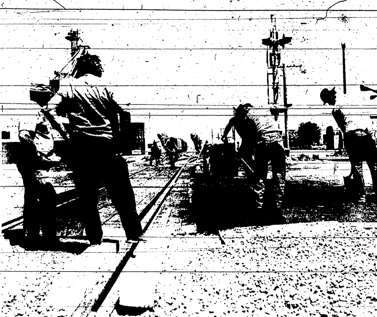
SMOOTHING out some of the trouble for Burley drivers are members of a Union Pacific track gang, repairing this crossing. The Burley City Council has repeatedly discussed the problem of rough crossings at meetings the past several months. Here, workers spread street surfacing material after placing planks between the rails.
