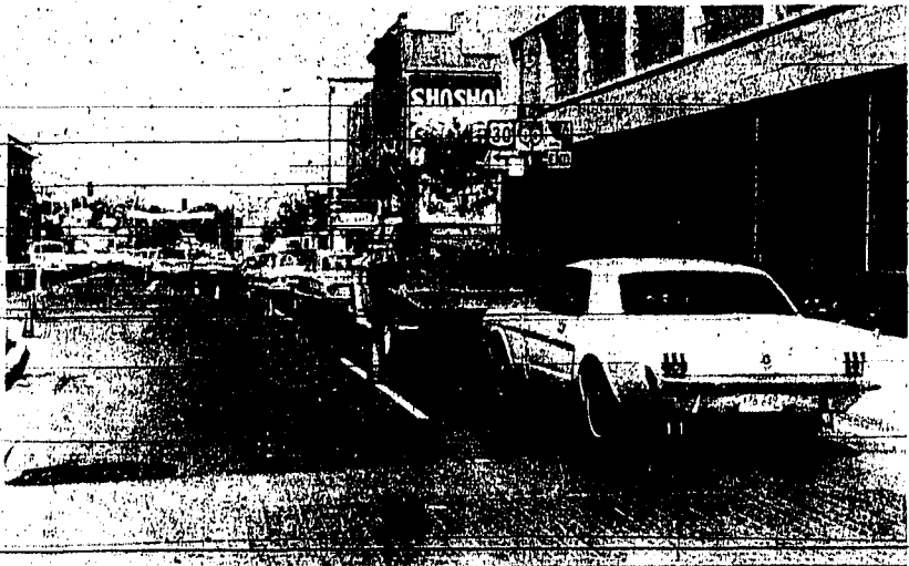
PAVING REPAIRS at the intersection of Shoshone Street and Main Avenue Tuesday caused traffic on Shoshone to be diverted into the lanes normally used by northbound vehicles, using one lane in each direction. The result was this long string of autos and trucks headed north, extending from Second Avenue North through the intersection of Main and Shoshone. This view was photographed about 4:15 p.m. Tuesday. The paving repairs were continuing today in the mall on Main Avenue.
