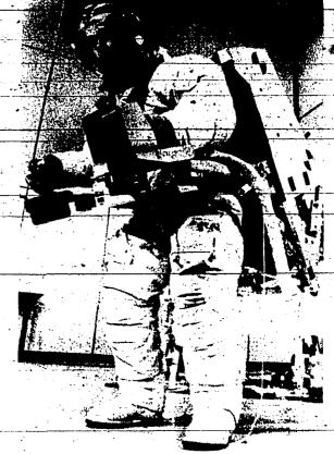
LATEST LOOK in spacesuits features a newly developed backpack housing a jet-powered unit which will permit weightless astronauts to maneuver inside a future Skylab, the projected orbiting space station. Astronaut Bruce McCandless tests controls of the powerpack which has a 30-minute flight capability.
