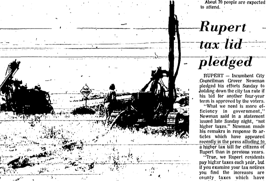
CONSTRUCTION crews have begun grading between Wendell and Tuttle for the next leg of Interstate 80N through that area of the Magic Valley. Here a driller prepares holes for blasting in a rocky stretch along the present Highway 25. Some grading and bridge work is now in progress.
