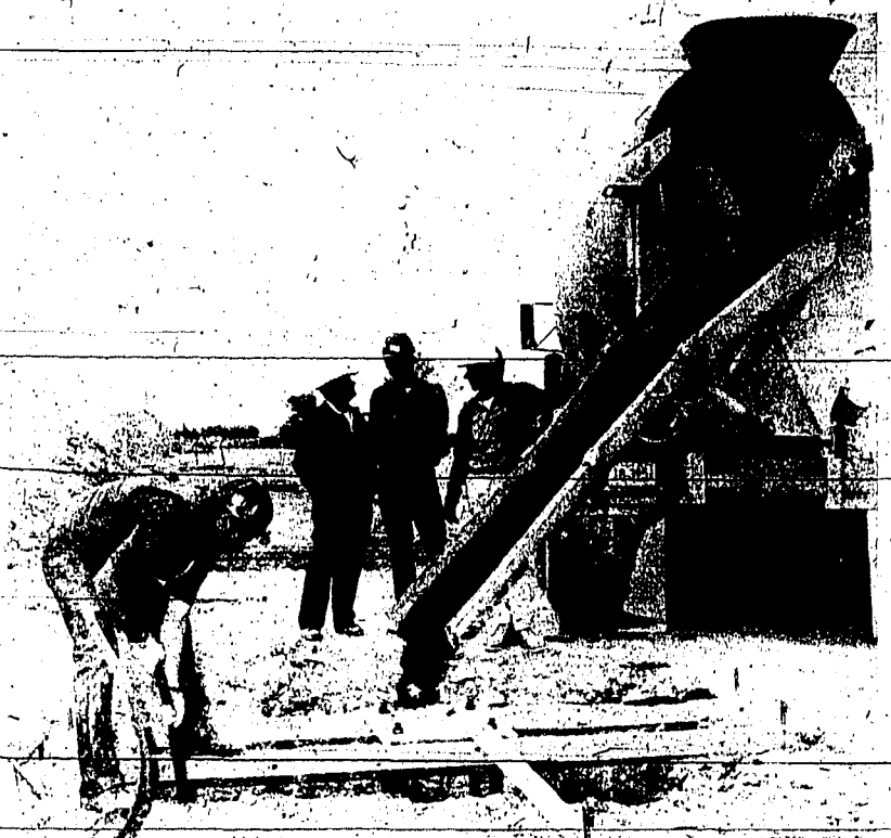
CONSTRUCTION CREWS poured concrete for footings at the site of the new Tupperware plant at the south edge of Jerome Tuesday. Building of the plant is moving ahead rapidly, although the project is still in its early phases. The plant is scheduled to be in production by mid-1972.
