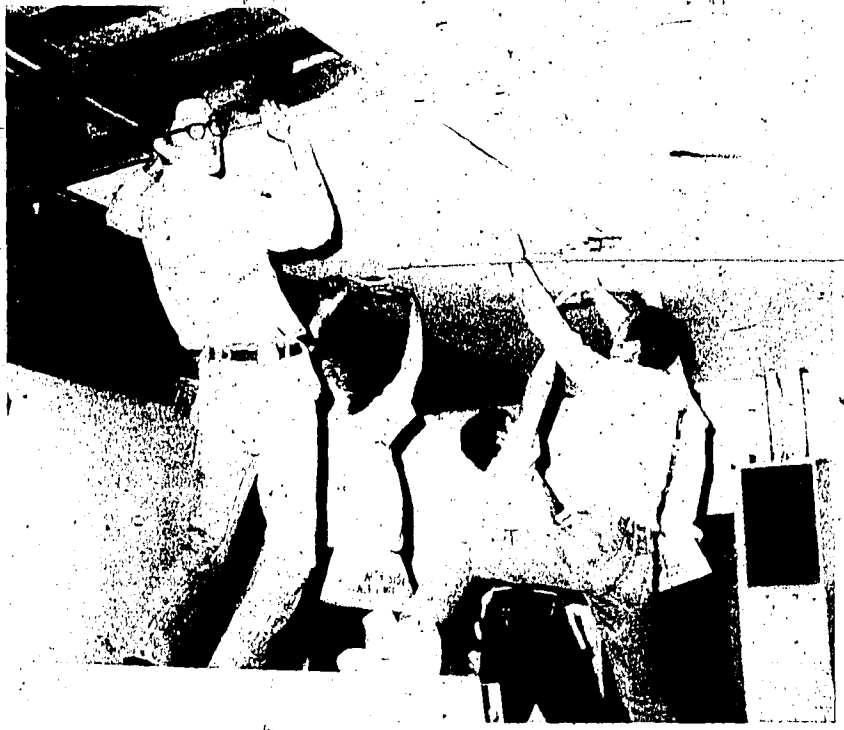
SEVERAL YOUNG, ambitious fellows give a helping hand as they lower the ceiling in the new HOPE building in Jerome. The organization will be open in its new location soon.
