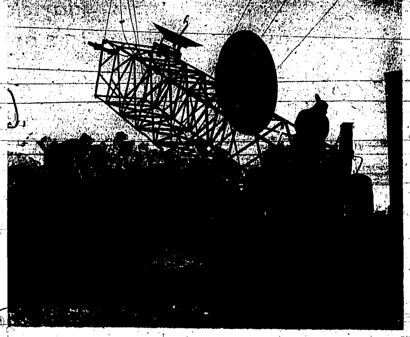
Crane lifts tower WINDS TOPPLED the Cable Vision tower on the butte north of Twin Falls Monday but service has been restored with the help of a giant crane, shown lifting the tower in above photo. The crane lifted the tower back into position and is holding it there until cement trucks can get into the muddy area to pour a new footing, probably today. At left, crews survey the estimated $1,000 damage and prepare to restore service to viewers in Twin Falls, Gooding, Jerome, Kimberly, Filer and Mountain Home.
