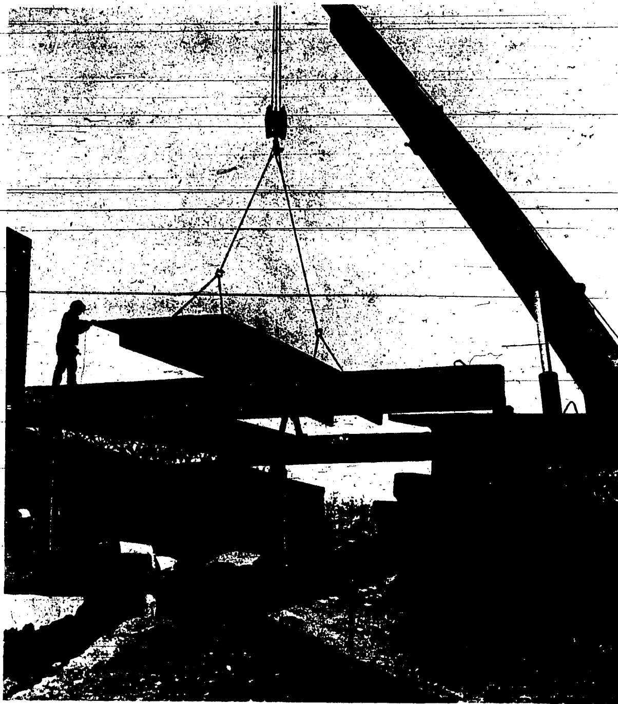
CONCRETE BEAM, weighing 15,000 pounds and representing several thousand dollars in community donations, is guided into place in the roofing structure of the new year-around swimming pool in Twin Falls. The building, at the north side of the YM-YWCA building on Elizabeth Boulevard, is progressing as rapidly as funds will permit.
