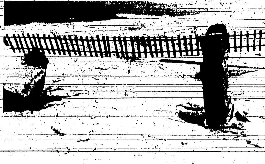
RAILROAD tracks hanging in the air mark spot where rain-swelled Corace River swept away a bridge during southern Italy's current rainstorms. Police say at least 14 persons have died in mudslides and flooding with thousands left homeless. (UPI)
