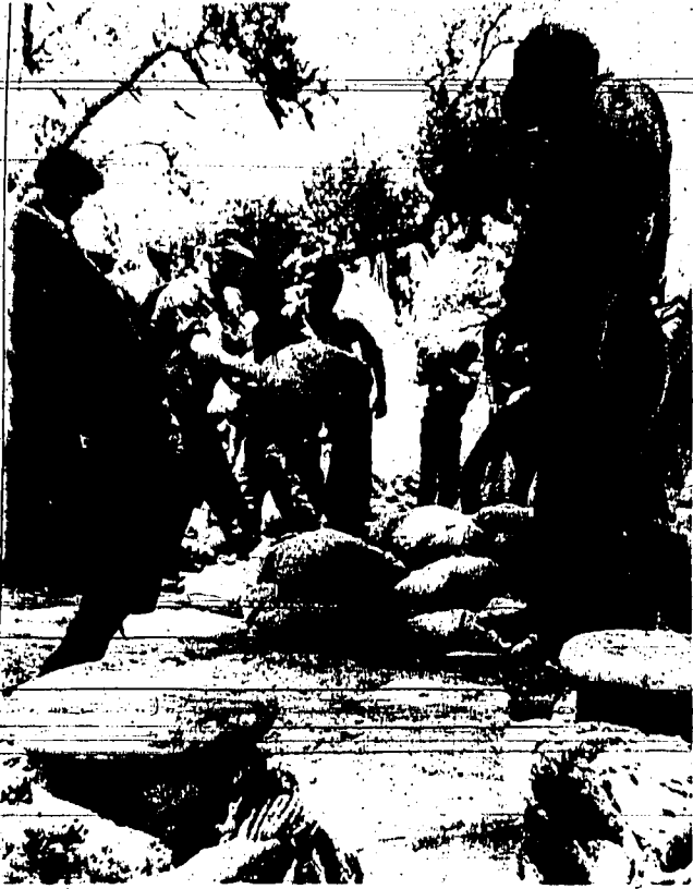
LOUISIANA National Guard Infantrymen from Jonesboro do their groundpounding loading sandbags aboard barges at the Army Corps of Engineers Bayou Foule Docks. The barges, covered with sand bags are to be kept ready in case of levee break. Floodwaters from the Mississippi in the Atchafalaya Basin toward Morgan City endangering its levees. (UPI)
